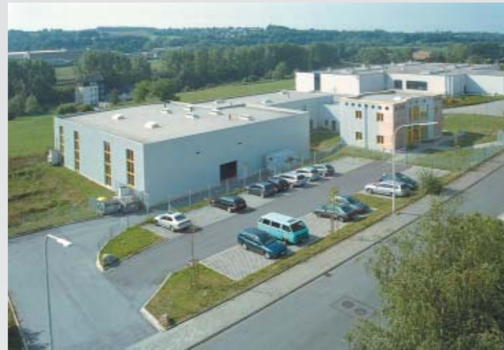
Our company buildings in Wuppertal-Vohwinkel
